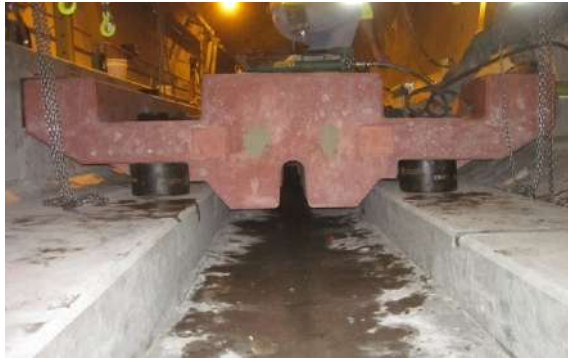
Sound Transit – High Density Floating Slabs
